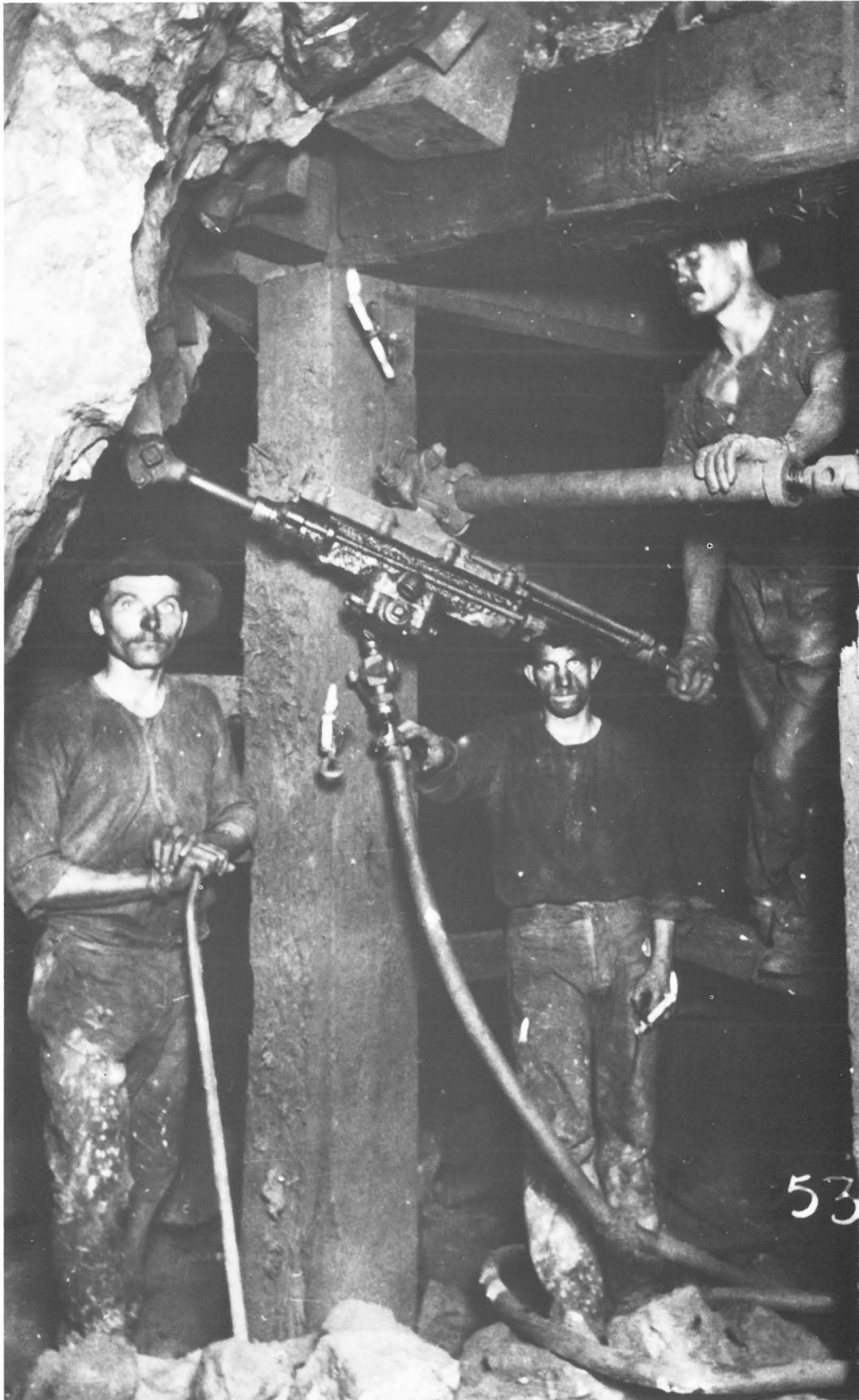
Drilling a round in a square-set stope, Warren district, c. 1910. Courtesy of Bisbee Mining and Historical Museum.
