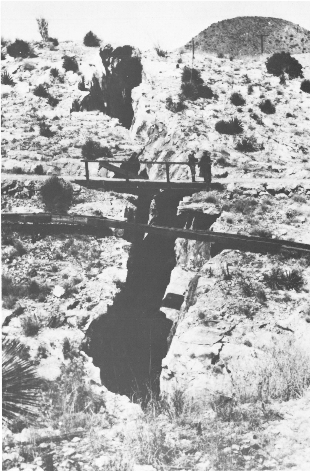
Subsidence crack resulting from sulfide oxidation and reopened by mining, Warren district. Courtesy of Bisbee Mining and Historical Museum.
