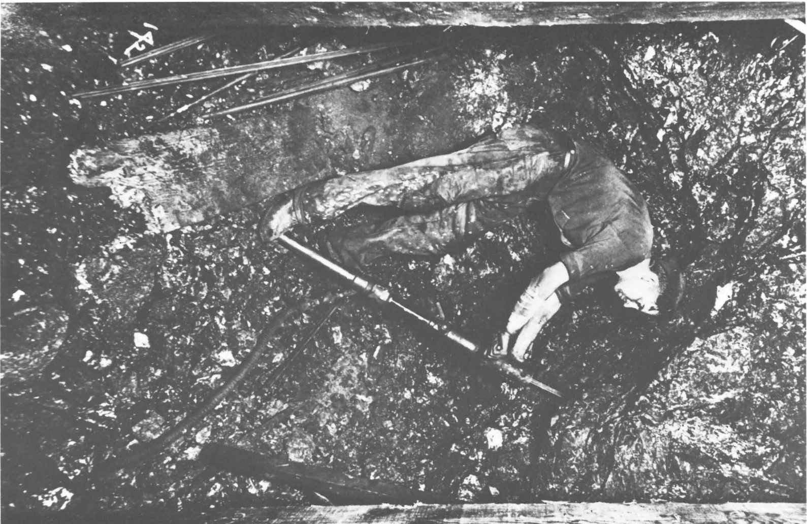
Drilling in a stope of oxidized ores, 1908. Courtesy Bisbee Mining and Historical Museum.
