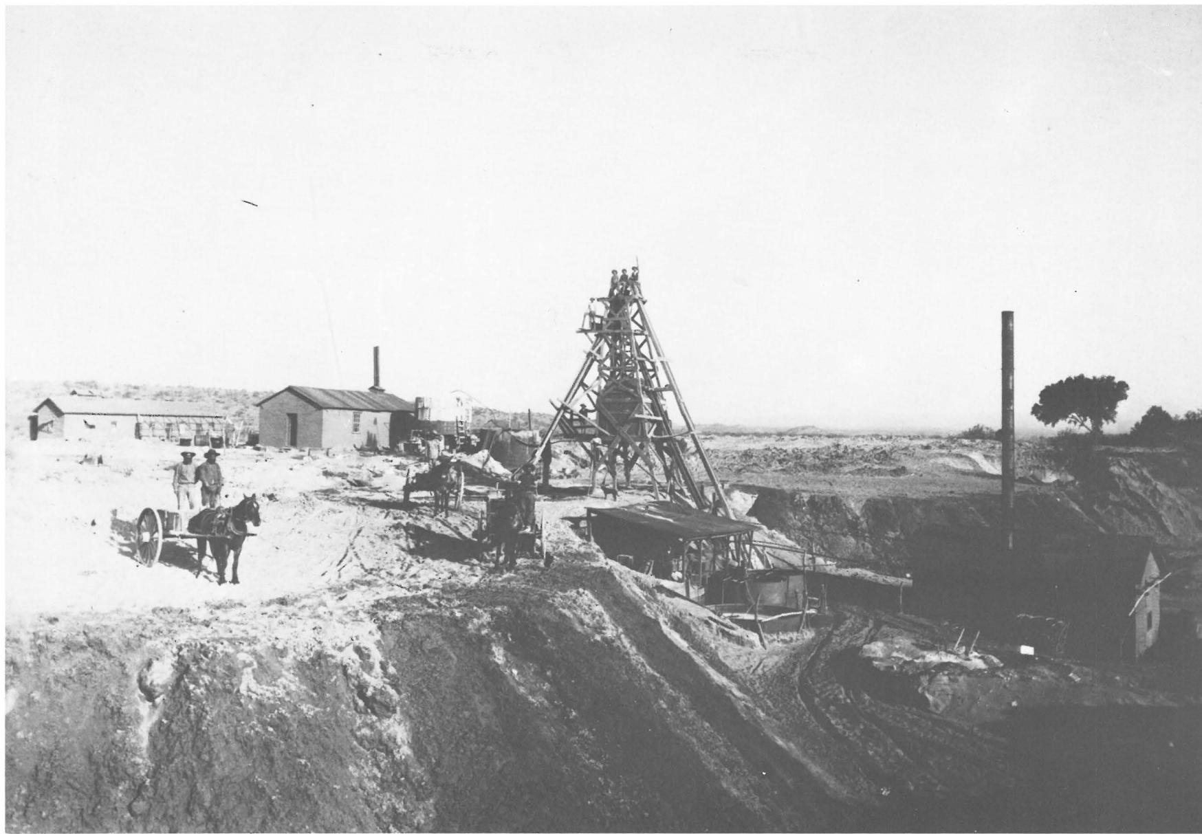
Reportedly first commercial application in United States of cyanide leach to mine tailings. Vulture mine, c. 1892. Courtesy of the Arizona Historical Society/Tucson.
