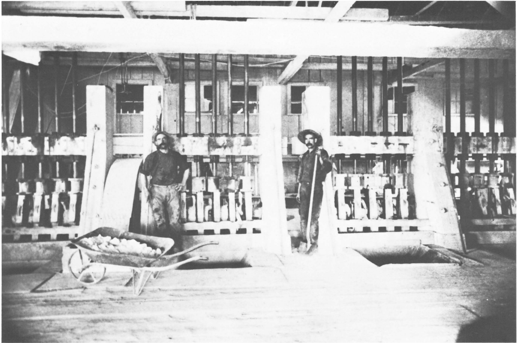
Stamp mill at Pinal City treated ore from the Silver King mine. c. 1882. Courtesy of the Arizona Historical Society/Tucson.
