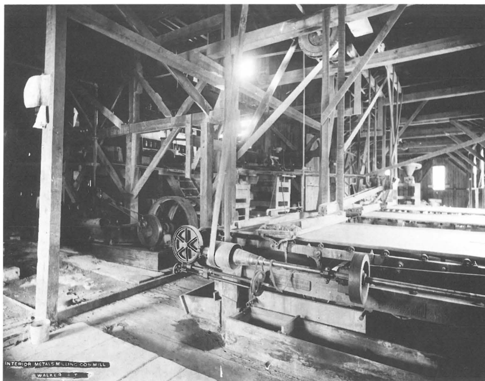
Interior view of mill operated by the Metals Milling Co. Gravity tables in right foreground. Courtesy of Frank M. Murphy, III.
